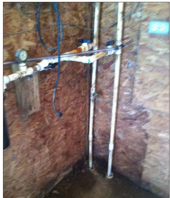
Figure 1. Three-quarter-inch supply line may restrict water supply to drinkers and cool cells.
