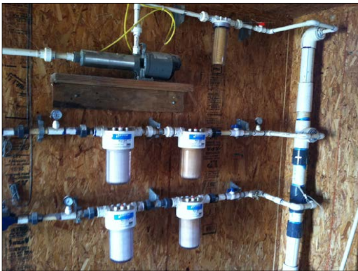
Figure 2. Four-inch supply line from well (upright pipe) with 1-inch drinker lines (brood and off end) and cool cell line (above) coming off of it.
