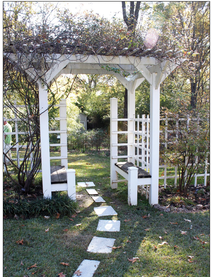
This arbor at the Eudora Welby House in Jackson, Mississippi, was originally made of wood, but the current structure was made primarily of metal to increase longevity and reduce maintenance costs. Material choices and budgetary challenges are just a few of the many complex issues that arise in efforts to preserve historic landscapes.
