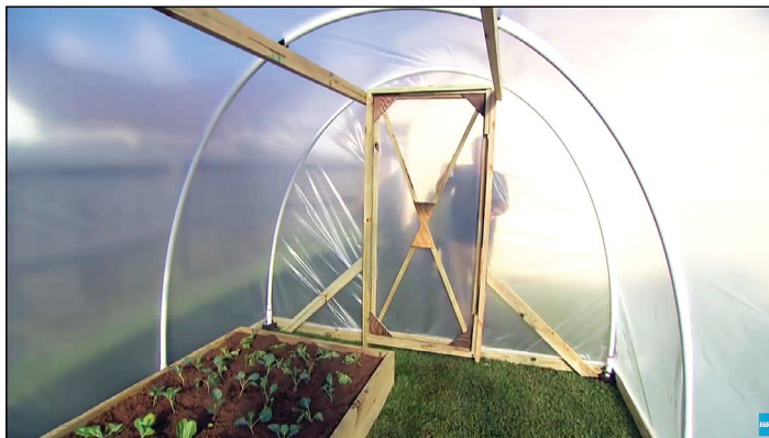
Step 10: Install the doors.
