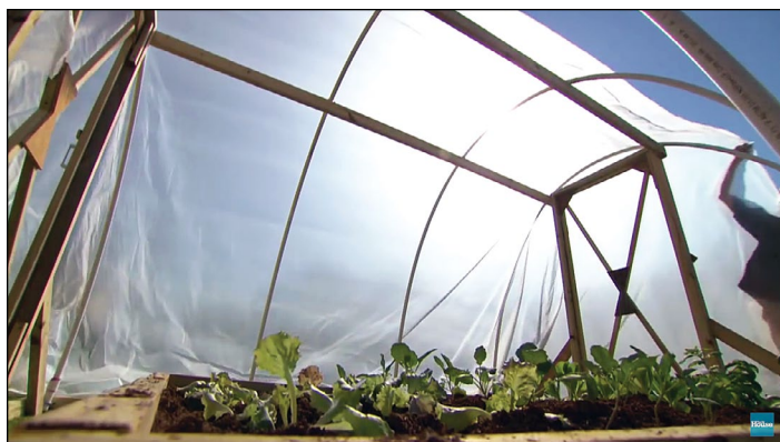
Step 11: Pull the plastic sheeting over the completed frame and secure it to the 2X4-inch base using screws or heavy-duty staples.
