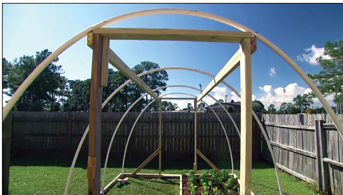
Step 9: Install the doorframe and 12-foot cross member for stability and support.
