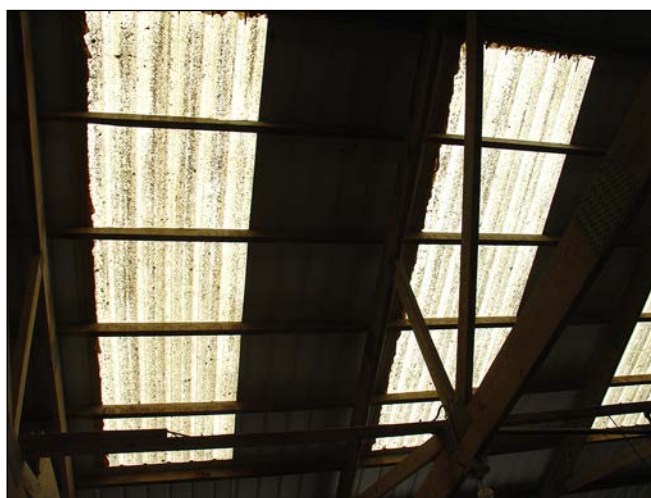
Figure 19. Translucent roof panels (skylights).
