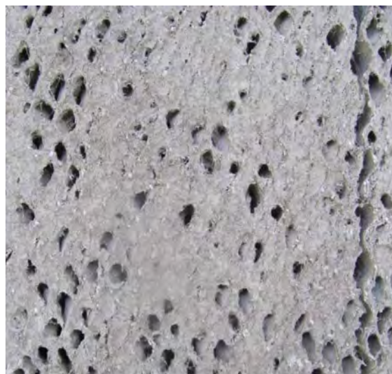
Figure 3. Mineral buildup clogs cool cell pads.
