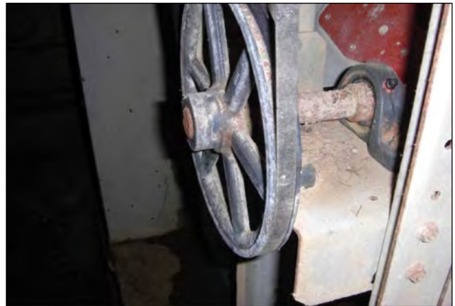
Figure 2. Belt-drive fans have bearings and grease fittings that need grease twice a year.
