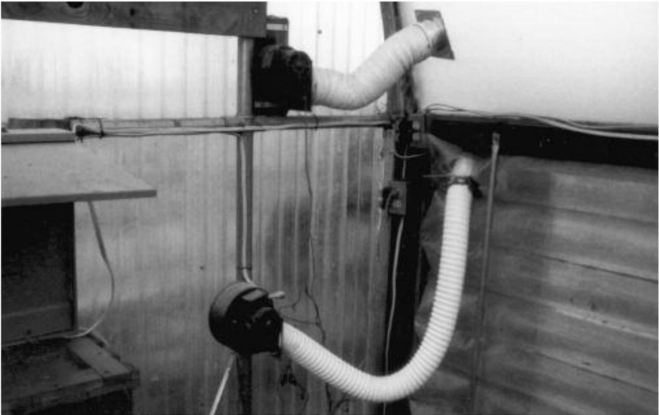
Small squirrel-cage blowers (1/4 or 1/2 HP) can be used to inflate between the two layers of plastic covering the greenhouse. It is important to use outside air for this purpose so that condensation does not collect between the layers.
