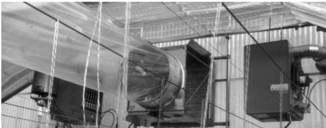
Traditional fan jet systems are commonly used to distribute heat produced by heaters and to recirculate inside air when the heating system is not in use.
