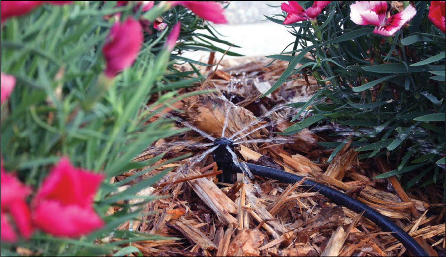
Figure 1. An adjustable micro-emitter sprinkler is irrigating a landscape bed of Telstar dianthus. (All photos by Gary R. Bachman)
