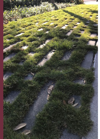
Figure 5 and 5-1. Maximize the use of pervious pavements. Grass is usually only suitable in between pavers when a soil is engineered to retain nutrients and appropriate moisture. The use of “grass-crete” is not recommended for high-traffic areas without irrigation and proper maintenance.
