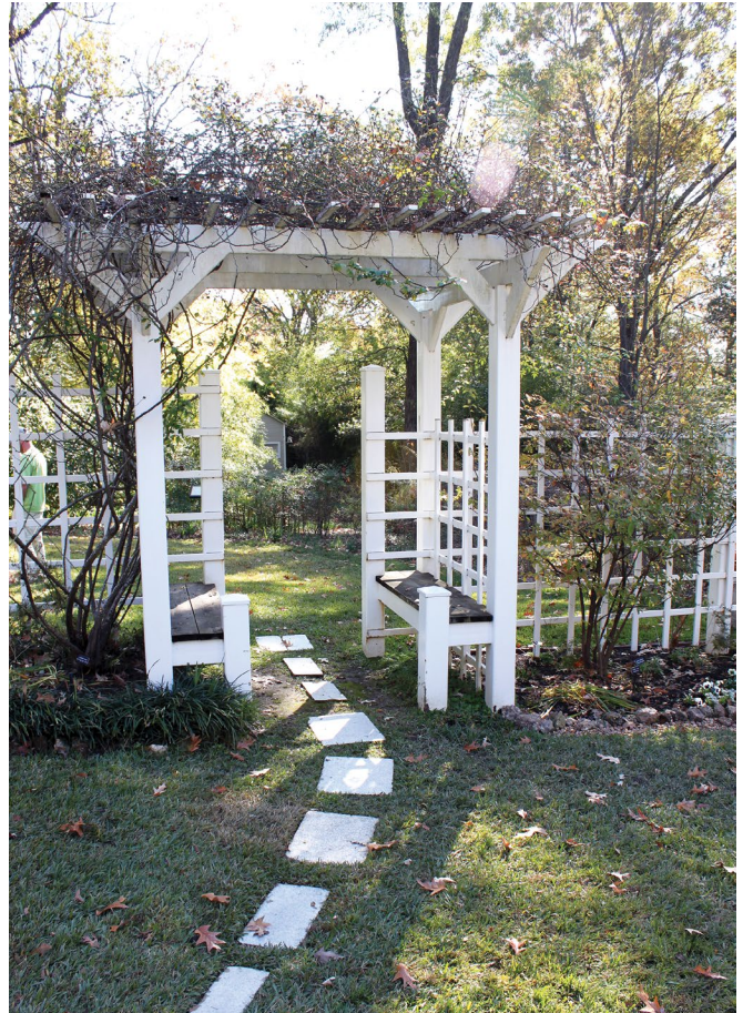
This arbor at the Eudora Welty House in Jackson, Mississippi, was originally made of wood, but the current structure was made primarily of metal to increase longevity and reduce maintenance costs. Material choices and budgetary challenges are just a few of the many complex issues that arise in efforts to preserve historic landscapes.
