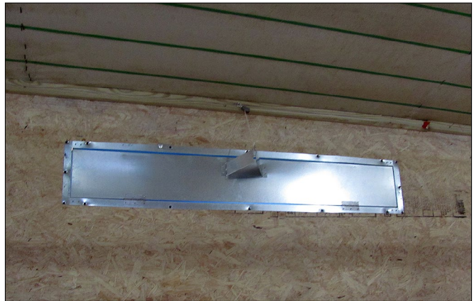
Figure 5. Sidewall air inlet.
