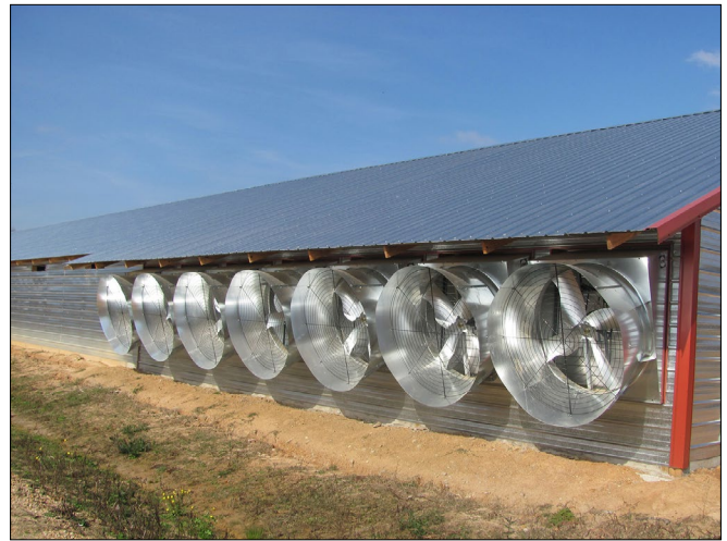
Figure 4. Fans in a broiler house.
