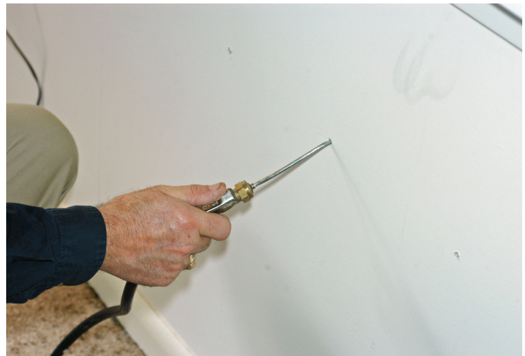
Figure 9. Insecticide foam. Insecticide-laced foam is injected into voids suspected of harboring termites.
