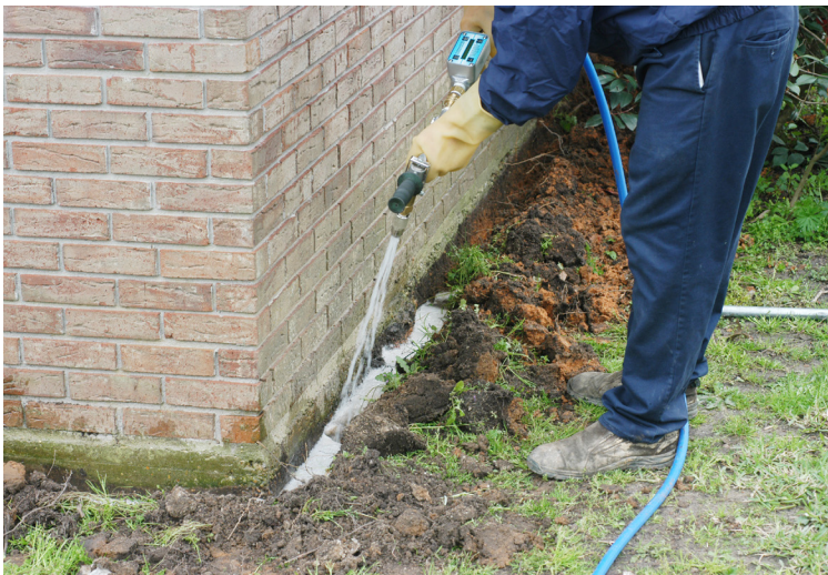
Figure 8. Soil-applied liquid termiticide. Liquid termiticide is applied to the soil around the building to create a barrier of treated soil through which termites have to travel to get into the building.
