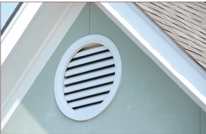
Gable vents with missing or torn screens allow easy entry for overwintering lady beetles, paper wasps, and other insects.
