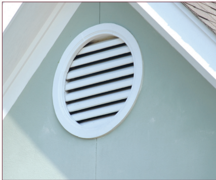
Gable vents should be screened with a layer of heavy hardware cloth and a layer of insect-proof window screen.
