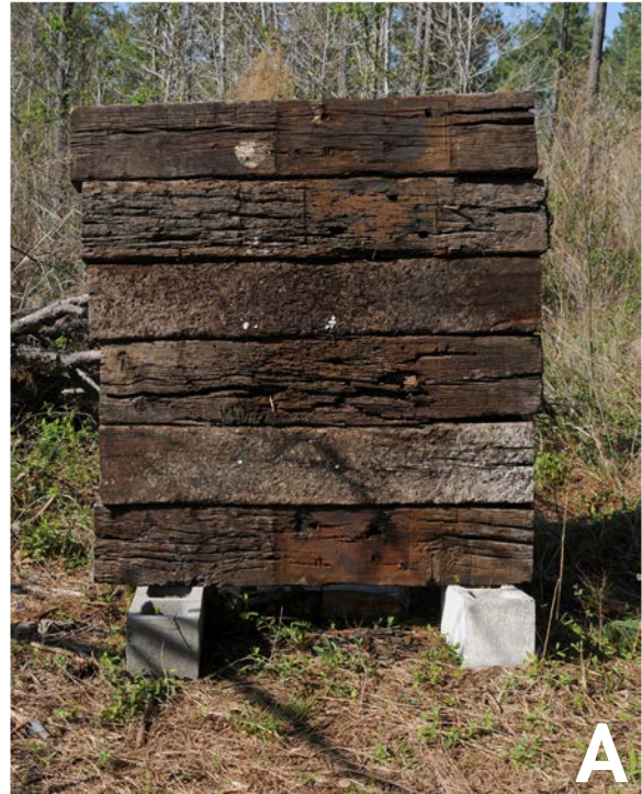
Space the left and right cinder blocks according to the width of the backstop you are constructing.
