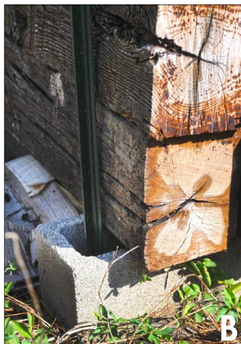
Next, drive the T-posts into the back left and right cinder blocks. These T-posts provide support for the crossties as they are stacked.
