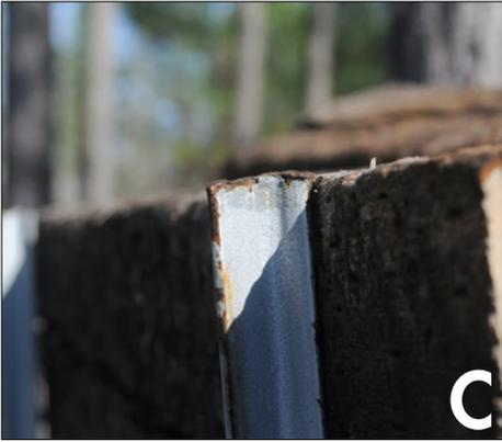
The T-posts should be level with the back of the top layer of crossties once the structure has been constructed. This is to prevent any ricochet from a projectile striking the metal of the T-post.
