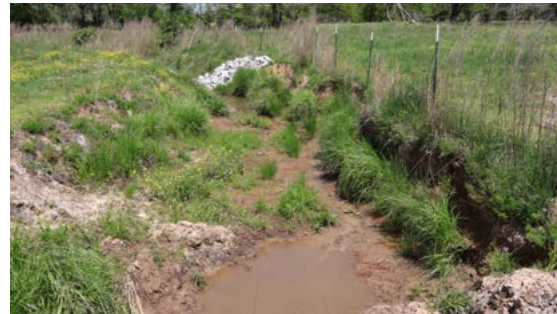
Figure 3B. Fence exclusions, check dam rock structure, and streambank protection.
