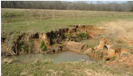
Figure 3A. Ditch and culvert drainage caused severe land erosion.
