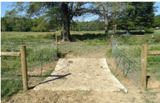
Figure 7. Fence exclusion and concreted heavy-use-area protection of a watershed stream.
