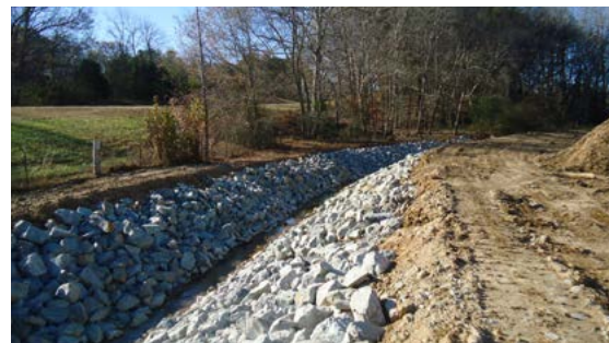
Figure 4B. Streambank protection using rock structures.
