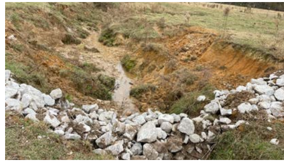
Figure 5B. Check dam rock structure.
