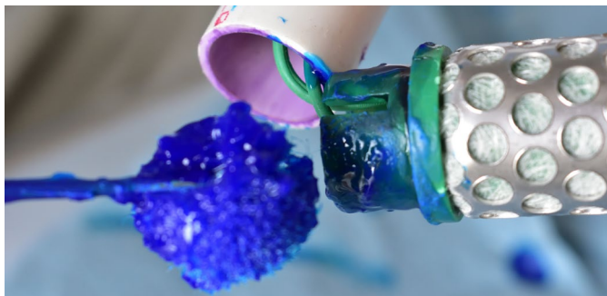
Figure 3.16. Apply ABS-PVC cement to the sensor collar.
