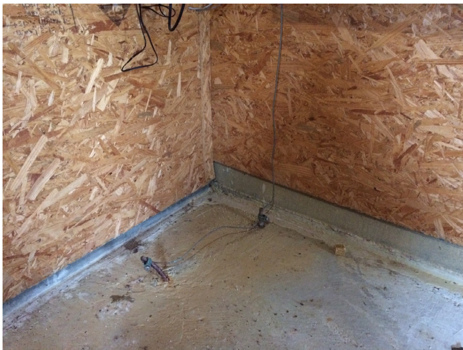
Figure 2. A Ufer ground is achieved by bonding the steel rebar on the left side of the picture to the ground rod on the right side. The rebar in this picture is reinforcing the concrete. Ufer grounds are a good way to reduce resistance and improve an overall electrical grounding system.
