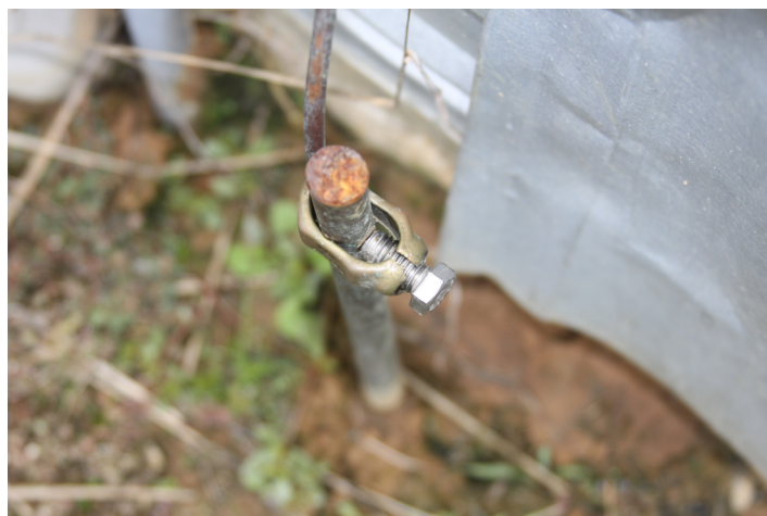
Figure 3. Broken clamps can increase resistance due to a poor connection. This problem should be corrected immediately. Inspecting ground wires, clamps, and rods yearly is a good idea.
