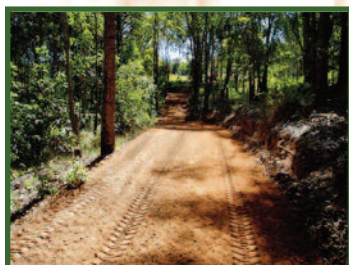
Fire Lane Construction - a monitored forest management practice Photo: www.totalearthworks.com
