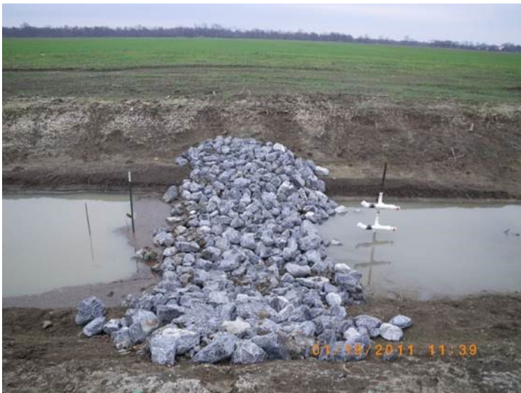
Figure 14. A low-grade weir made of riprap covering an earthen berm. The structure was monitored for water quality improvements on a working farm in the Mississippi Delta.
