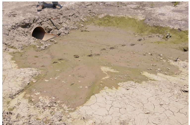
Figure 8. A slotted inlet pipe beneath a levee for grade stabilization and erosion control in the Mississippi Delta.
