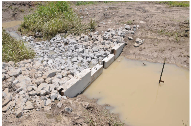
Figure 13. An interlocking, prefabricated low-grade weir reinforced with riprap retaining water on a working farm in the Mississippi Delta. Photo by Austin Omer.
