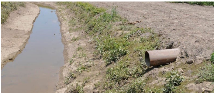
Figure 2. The image on the left shows the outflow of a slotted inlet pipe where it exits through an earthen berm or pad and discharges into a drainage ditch. The image on the right shows the slotted pipe intake installed at the edge of a crop field to receive runoff.
