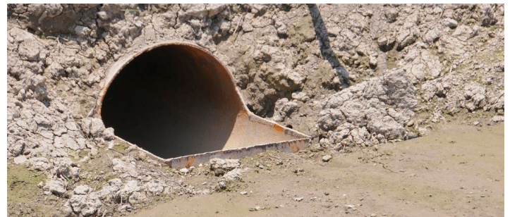
Figure 2. The image on the left shows the outflow of a slotted inlet pipe where it exits through an earthen berm or pad and discharges into a drainage ditch. The image on the right shows the slotted pipe intake installed at the edge of a crop field to receive runoff.
