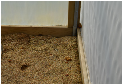
Figure 3. Wooden foundation with pea gravel.
