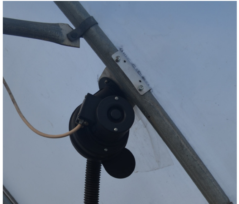
Figure 13. A squirrel-cage blower (fan) is used to inflate between the two layers of plastic covering the greenhouse.
