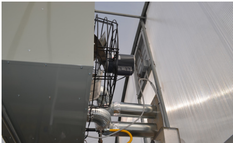
Figure 8. Heater intake (bottom) and exhaust (top) ducts leading from and to the outside.
