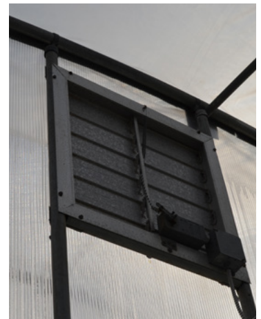
Figure 9. A top ventilation fan and top intake louver provide ventilation for humidity and early temperature control.
