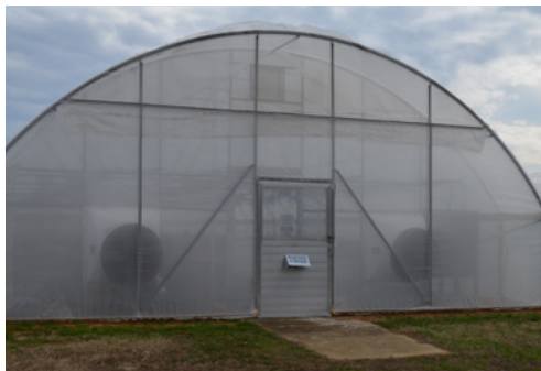
Figure 5. Insect-screened area on the front of a greenhouse; it is also used as a double entry.
