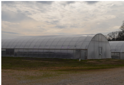
Figure 2. A Quonset-style greenhouse covered with double poly plastic and with a pressure-treated wood foundation.
