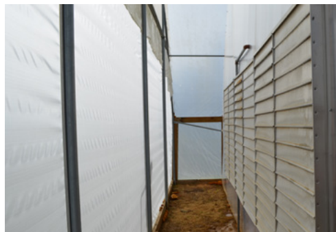
Figure 6. Insect-screened area on the back of a greenhouse.
