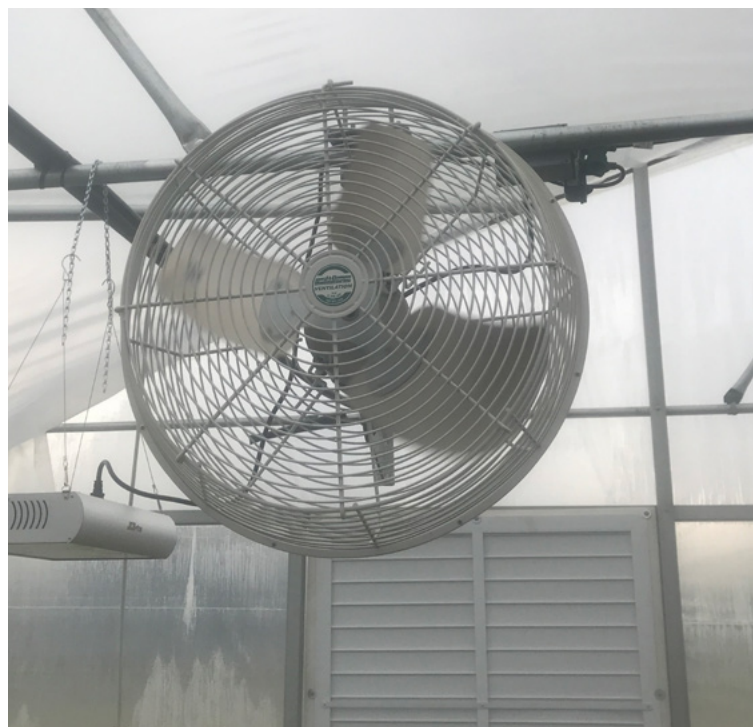
Figure 12. Horizontal fans provide air movement within the greenhouse.
