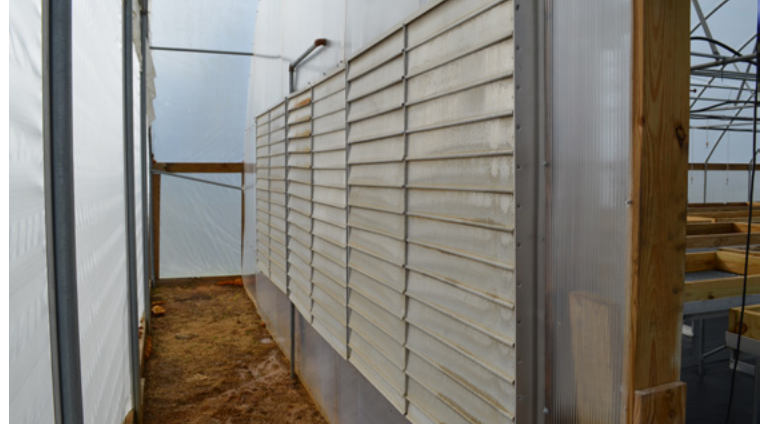
Figure 11. Intake ventilation louvers open to allow air movement through the greenhouse for temperature control.
