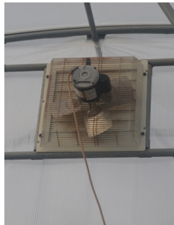
Figure 9. A top ventilation fan and top intake louver provide ventilation for humidity and early temperature control.
