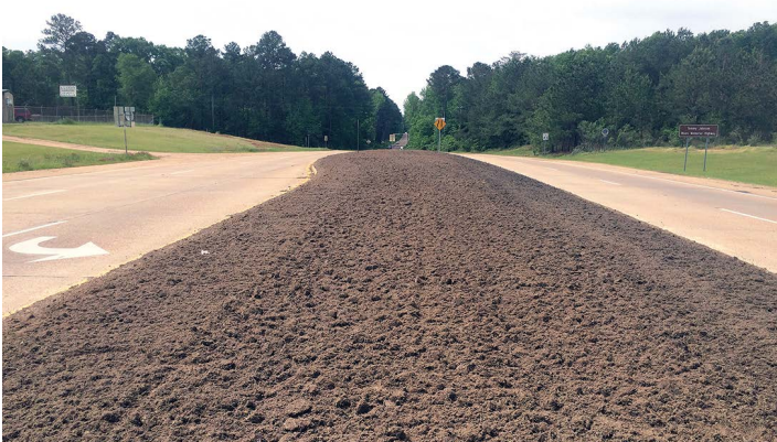
Figure 1. This elevated median was tilled before sowing. Multiple passes over a site may be required to break down large clods. A smooth soil surface prevents broadcast seed from getting buried too deep between clods during weathering.
