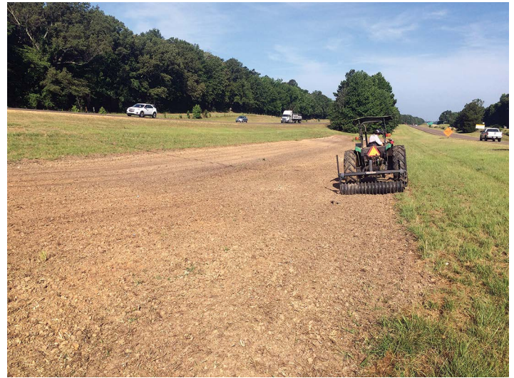
Figure 2. Cultipacking after seeding allows the seed to be pressed into the soil surface, allowing for greater seed-to-soil contact, which enables seed to absorb water and nutrients for germination and development.
