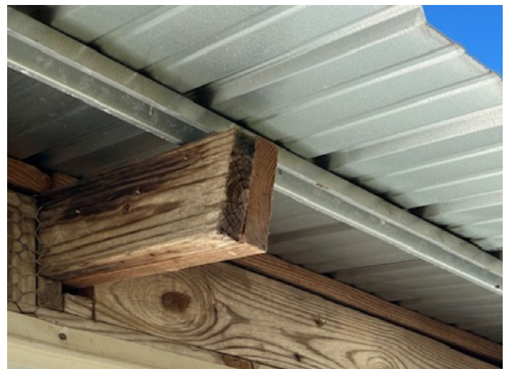
Figure 5. Replaced metal purling and truss tail repair.
