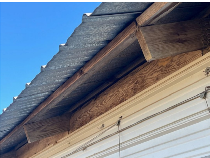
Figure 4. Traditional truss tail purling.
