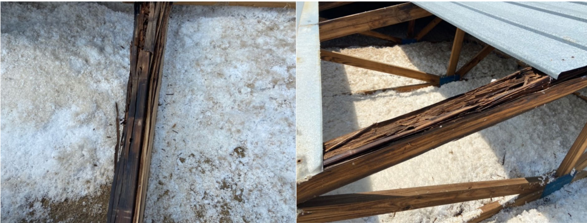
Figure 3. Rotten trusses from fastener leaks.
