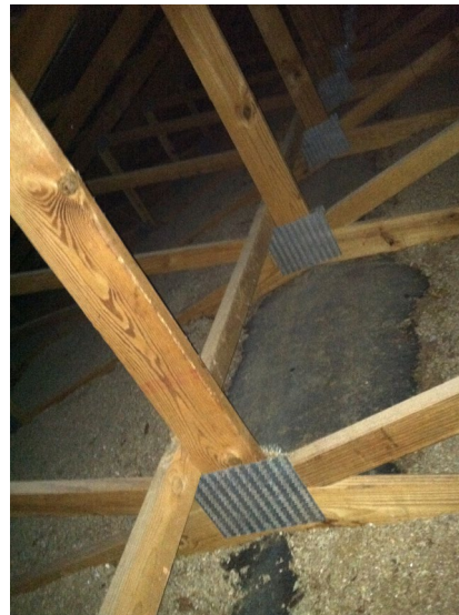
Figure 3. Uninsulated areas in an attic caused by settled insulation.
