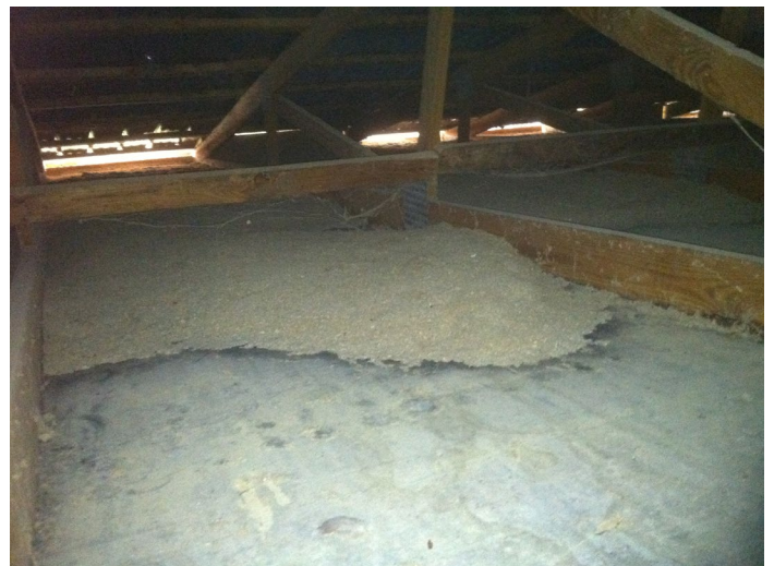
Figure 3. Uninsulated areas in an attic caused by settled insulation.
