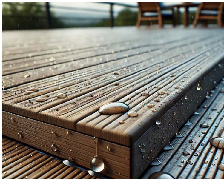
Figure 28. Wood-plastic composites, produced with solid and hollow cross-sections, are water resistant.
