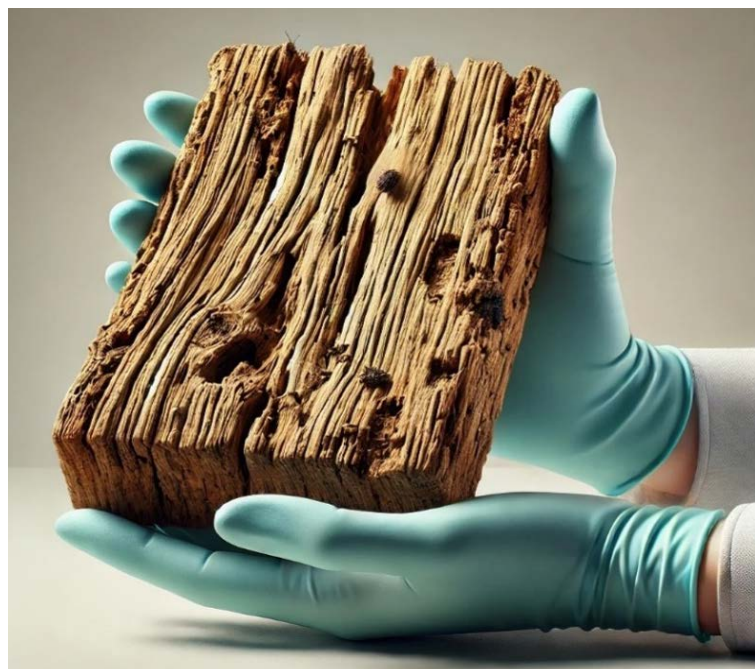
Figure 32. Comparison between non-decayed and decayed wood.
