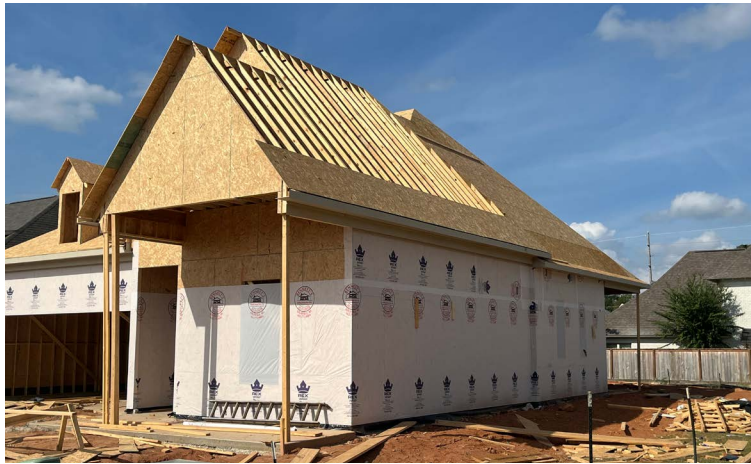
Figure 18. OSB is used for roof and wall sheathing to cover this home.
