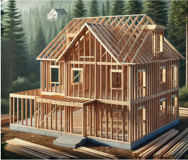
Figure 15. Wood framing with lumber as a traditional method for constructing residential houses.
