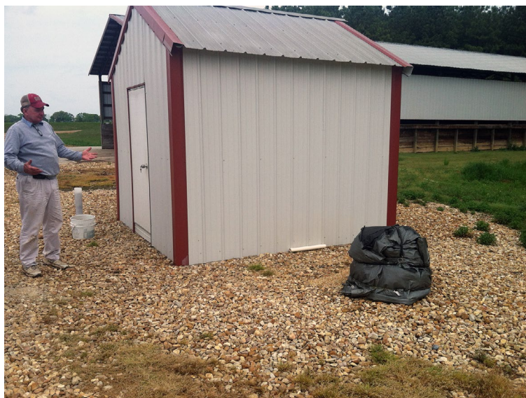
Figure 1. Many producers build some form of house over the well casing to protect it from the environment and other dangers.
