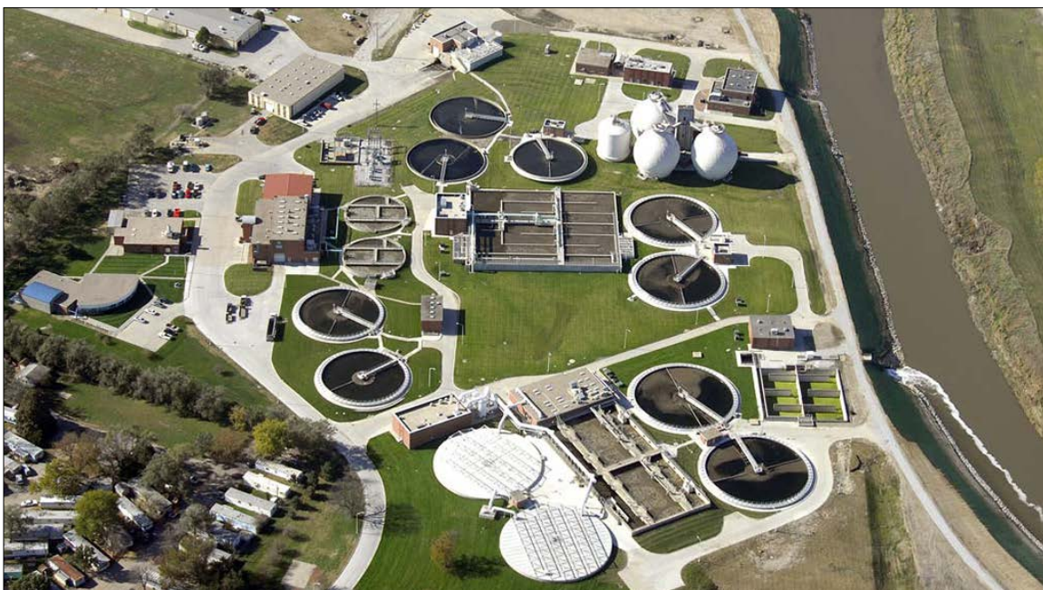
Figure 2. Theresa Street wastewater-treatment facility in Lincoln, Nebraska.
