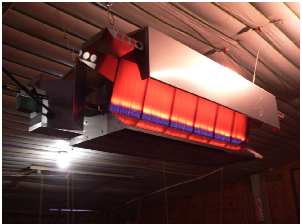
Figure 3. Rectangular open-flame radiant brooder. Photo credit: University of Kentucky, Biosystems & Agricultural Engineering.
