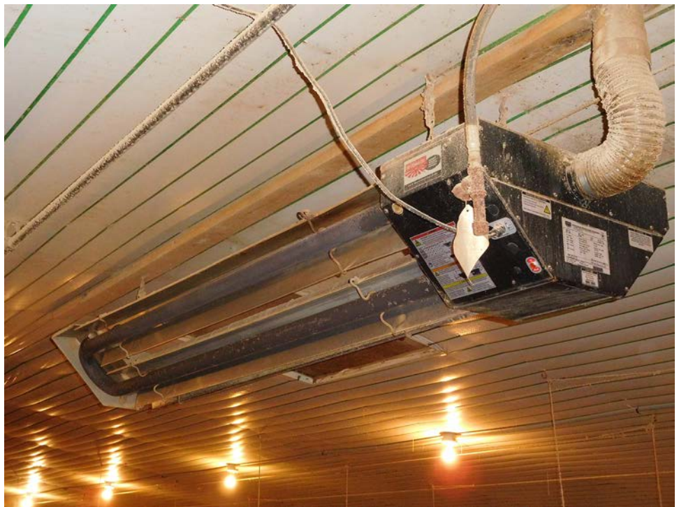
Figure 6. Closed-flame radiant tube brooder. Photo credit: University of Kentucky, Biosystems & Agricultural Engineering.
