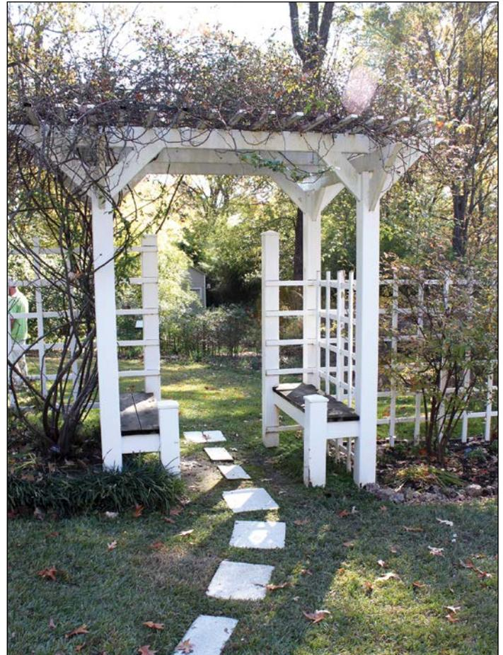
This arbor at the Eudora Welty House in Jackson, Mississippi, was originally made of wood, but the current structure was made primarily of metal to increase longevity and reduce maintenance costs. Material choices and budgetary challenges are just a few of the many complex issues that arise in efforts to preserve historic landscapes.
