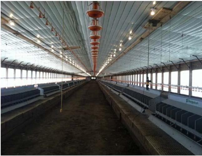
Figure 1. LED lights on 10-foot centers above the nests.
