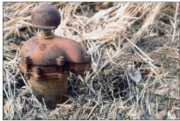
Figure 2. A vented well cap over the casing protects the water supply from surface water and other contaminants.
