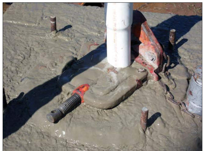
Figure 1. A cement and bentonite clay mixture around the well casing keeps surface water and pollutants from reaching the water supply.
