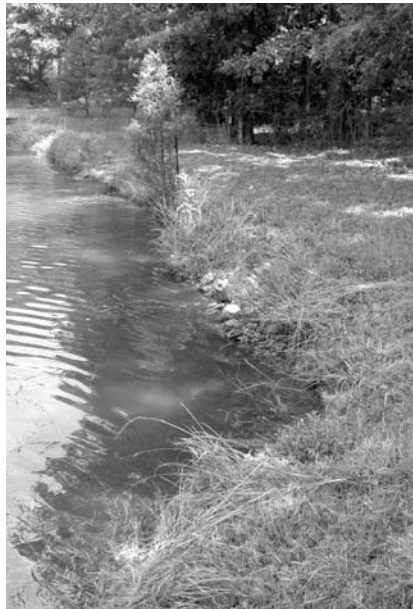
Mark eroded areas on pond banks
