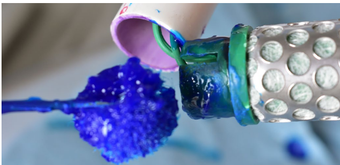
Figure 3.16. Apply ABS-PVC cement to the sensor collar.
