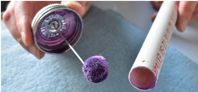
Figure 3.14. Apply PVC primer.
