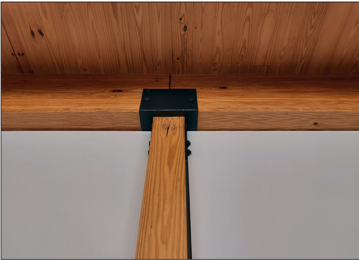
Figure 5. In the Auburn University Advanced Structural Engineering Lab, CLT was used for roofing (five-layer/ply, 10 feet in length). Glulam was used for the beams, and solid timbers were used for the framing. Unlike CLT—in which layers of several pieces of lumber are glued to produce a layer and then layers are joined in a 90-degree, cross-oriented fashion—Glulam is made of pieces of lumber laid in the same direction and then joined. Solid timbers are single pieces of wood and are not engineered by joining several pieces. Therefore, the Structural Engineering Lab is an example of a mass-timber-constructed building, not a CLT-constructed one specifically.
