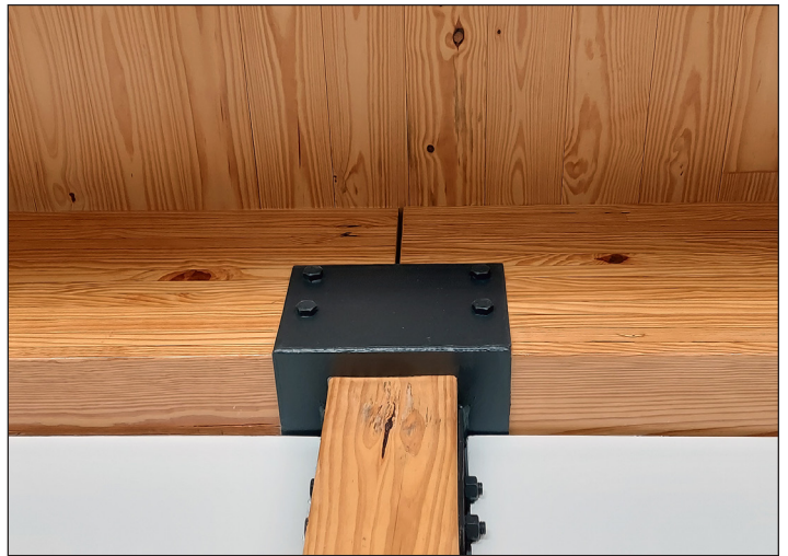
Figure 5. In the Auburn University Advanced Structural Engineering Lab, CLT was used for roofing (five-layer/ply, 10 feet in length). Glulam was used for the beams, and solid timbers were used for the framing. Unlike CLT—in which layers of several pieces of lumber are glued to produce a layer and then layers are joined in a 90-degree, cross-oriented fashion—Glulam is made of pieces of lumber laid in the same direction and then joined. Solid timbers are single pieces of wood and are not engineered by joining several pieces. Therefore, the Structural Engineering Lab is an example of a mass-timber-constructed building, not a CLT-constructed one specifically.
