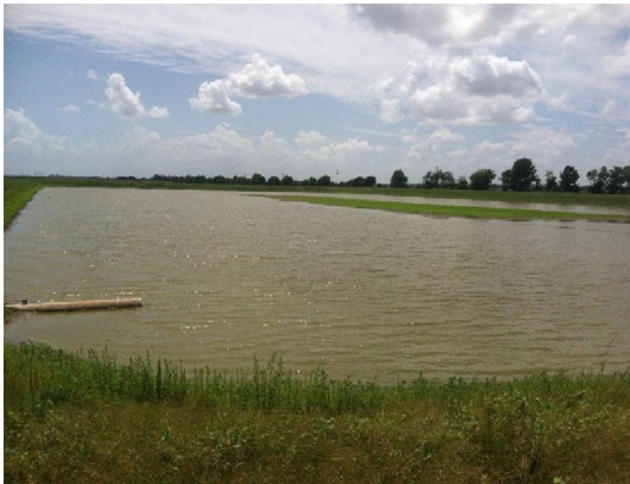
Figure 6. Bottom of an on-farm storage reservoir (approximately 10-acre surface area).
