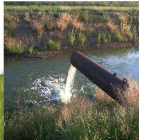
Figure 3. Left: Receiving end of a riser board pipe. The boards slide along the grooves in the front of the pipe, which keeps water from entering the pipe. Middle: Diagram of water flowing from a corn field on the left through a riser board pipe and into a TWR ditch. Notice the pipe is installed underneath a dike (pad). Right: Water flowing from a riser board pipe into a TWR ditch.
