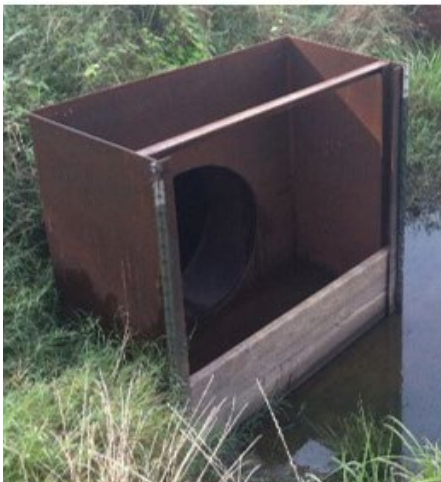
Figure 3. Left: Receiving end of a riser board pipe. The boards slide along the grooves in the front of the pipe, which keeps water from entering the pipe. Middle: Diagram of water flowing from a corn field on the left through a riser board pipe and into a TWR ditch. Notice the pipe is installed underneath a dike (pad). Right: Water flowing from a riser board pipe into a TWR ditch.
