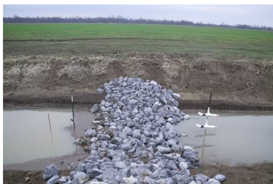
Figure 17. Low-grade weir made of riprap covering an earthen berm. The structure was being monitored for water-quality improvements on a working farm in the Mississippi Delta. Photo credit: Beth Baker
