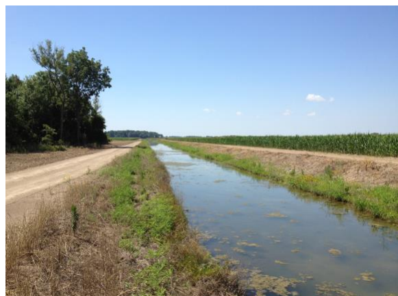
Figure 19. Full tailwater recovery ditch in the Mississippi Delta. Photo credit: Austin Omer
