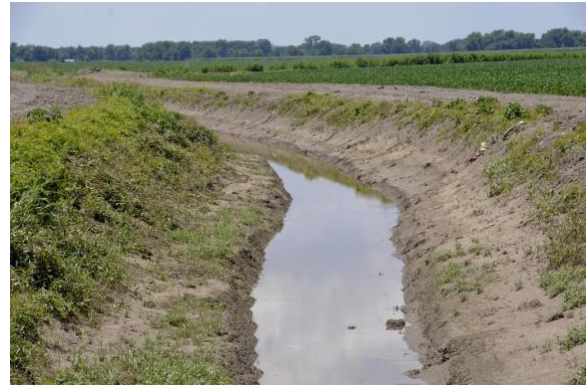
Figure 14. A drainage ditch that has undergone construction to widen the channel and create floodplain benches to create a two-stage ditch. Photo credit: REACH program
