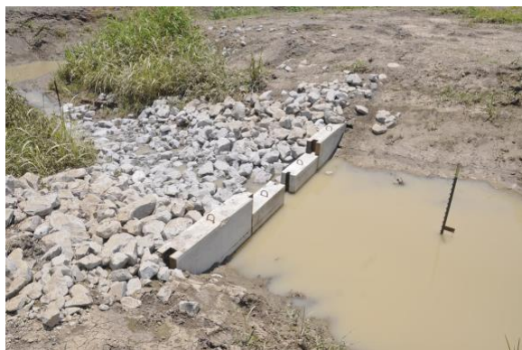
Figure 16. Interlocking, prefabricated, low-grade weir reinforced with riprap retaining water on a working farm in the Mississippi Delta. Photo credit: Austin Omer
