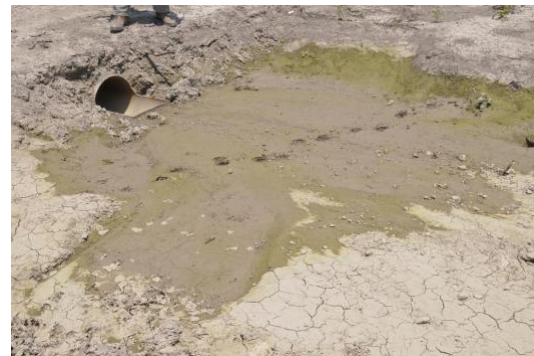
Figure 13. Slotted inlet pipe beneath levee for grade stabilization and erosion control in the Mississippi Delta. Photo credit: REACH program
