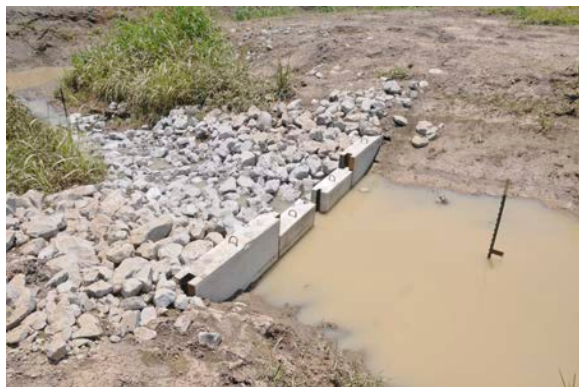
Interlocking, prefabricated, low-grade weir reinforced with rip-rap retaining water on a working farm in the Mississippi Delta. Photo credit: Austin Omer
