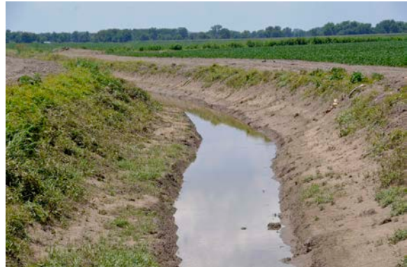
A drainage ditch that has undergone construction to widen the channel and create floodplain benches to create a two-stage ditch. Photo credit: REACH program
