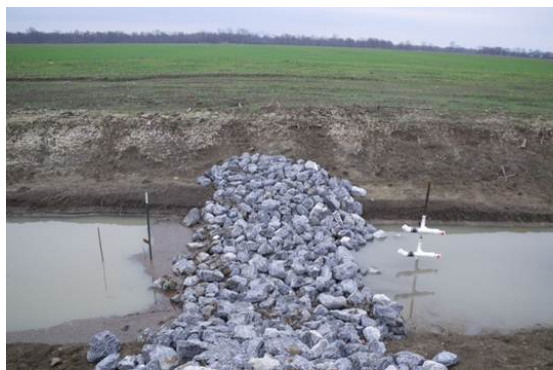
Low-grade weir made of riprap covering an earthen berm. The structure was being monitored for water-quality improvements on a working farm in the Mississippi Delta. Photo credit: Beth Baker
