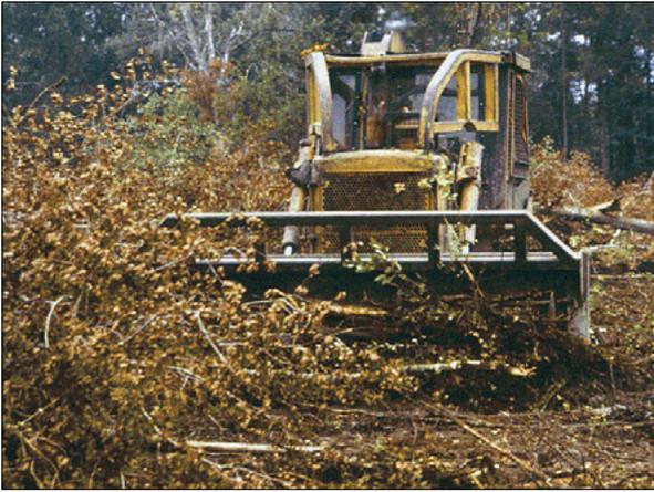
Figure 3. Once felled, debris is raked into piles or rows to complete the land-clearing operation.
