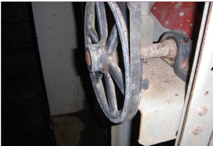
Figure 2. Belt-drive fans have bearings and grease fittings that need grease twice per year.
