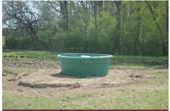
Placement of a trough on a concrete pad with soil erosion and pasture damage occurring around the base of the pad.
