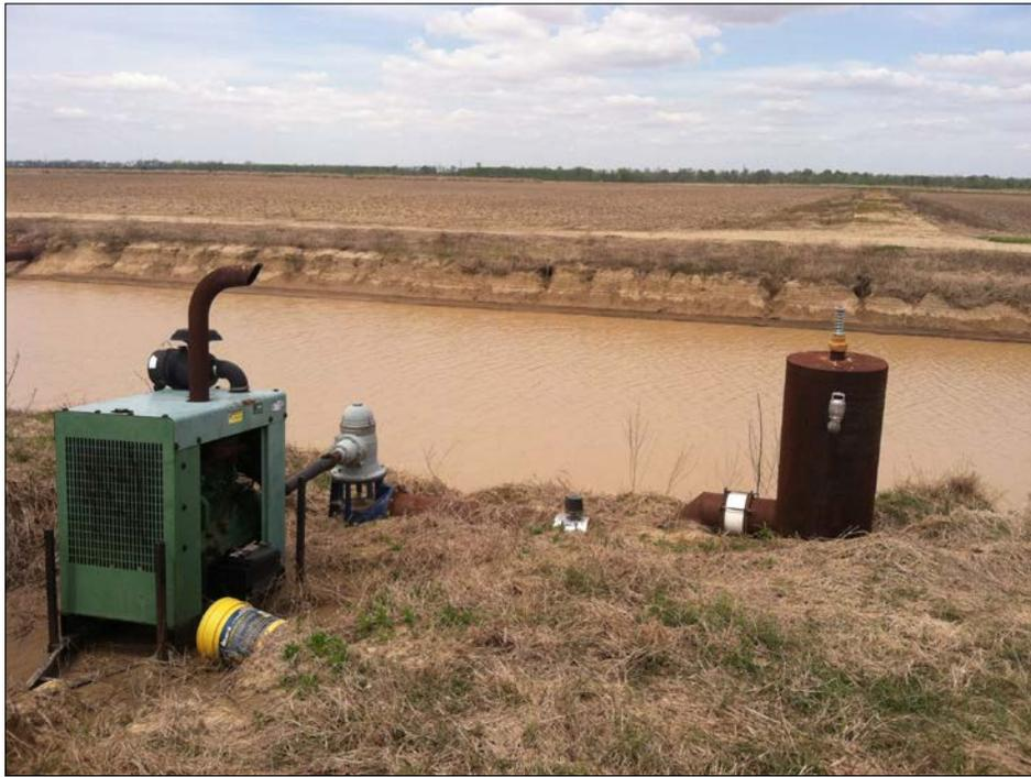
Figure 7. Surface water pumping plant used to irrigate water from the adjacent TWR ditch.
