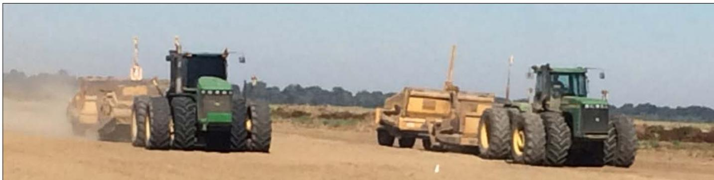
Figure 1. Tractors pull dirt pans and level land to create a TWR system in the Mississippi Delta.
