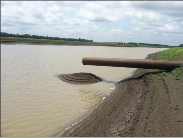
Figure 5. Large TWR ditch in the Mississippi Delta. Notice the sediment buildup as a result of runoff from the adjacent field.
