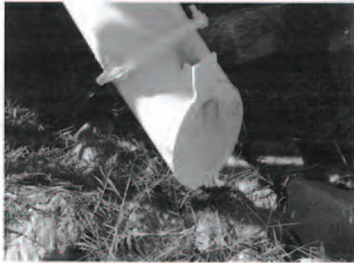
View of overflow pipe and flapper gate.
