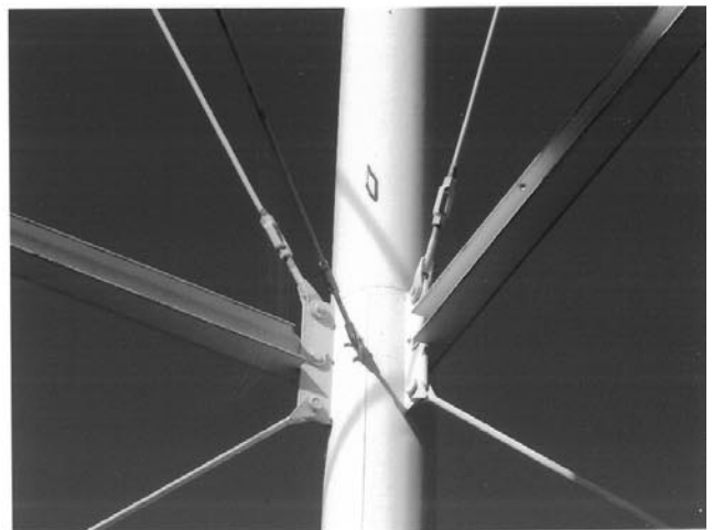
View of rods and struts.
