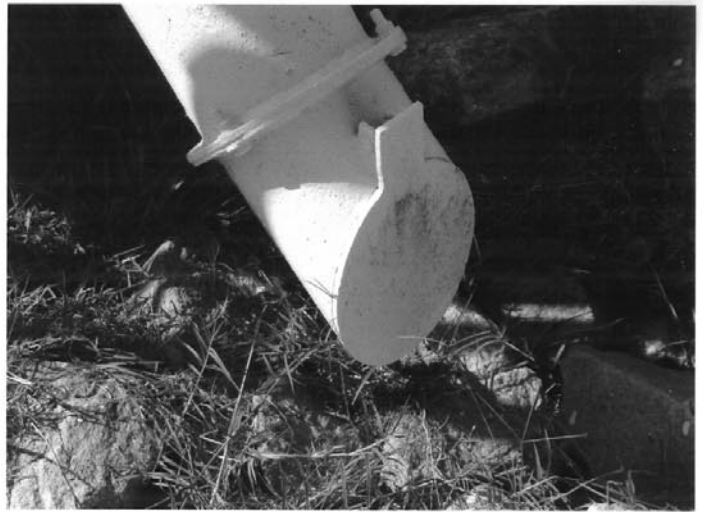
View of overflow pipe and flapper gate.
