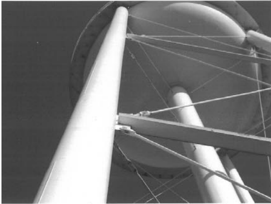
View of columns and exterior ladder.
