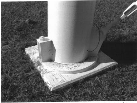
View of foundations, base plates, anchor nuts and bolts.
