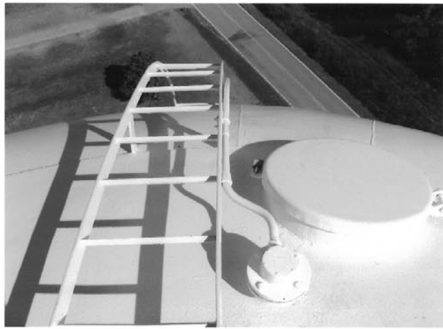
View of locked roof manway.
