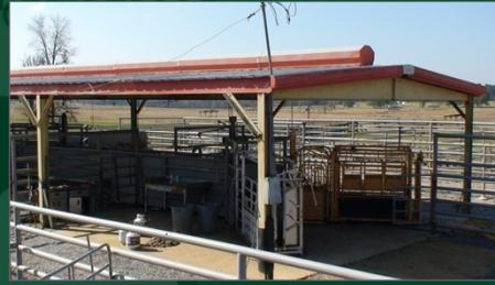
Covered handling facilities
