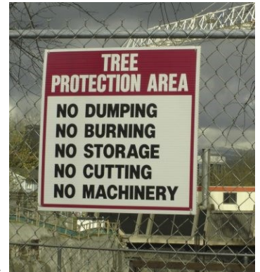
Using signs along with fencing will alert workers during construction. This will likely aid in protecting trees.
