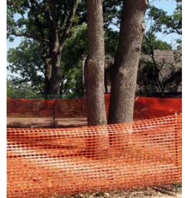
Construction fencing placed at the edge of the critical root area. There should be NO construction activities within this barrier.
